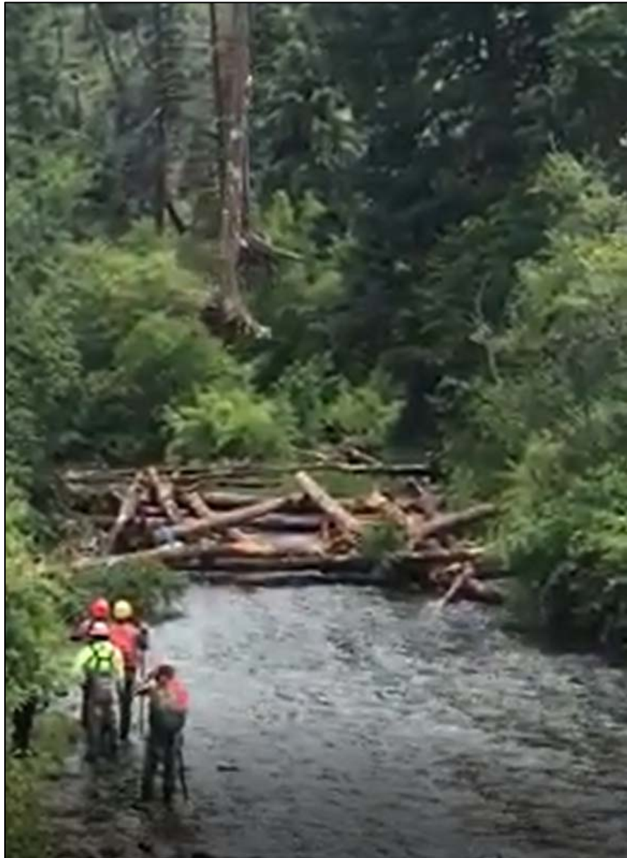
FIGURE 30 HELICOPTER LARGE WOOD PLACEMENT
