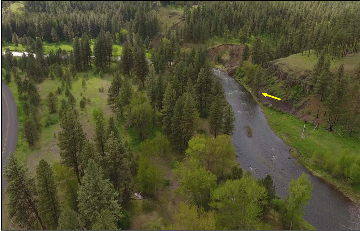
FIGURE 15 VIEWING UPSTREAM. STATIONING MC 22+00 – 26+00, SC2 ENTRANCE
