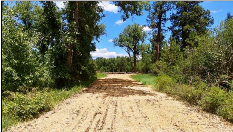
FIGURE 26 SEEDED AND MULCHED DECOMMISSIONED ROAD AT STATIONING MC 55+00
