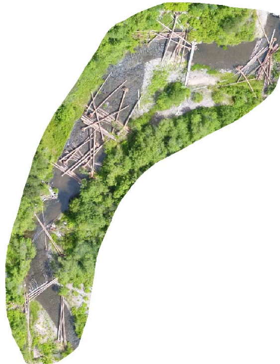
FIGURE 34 POST CONSTRUCTION DRONE ORTHOMOSAIC IMAGE
